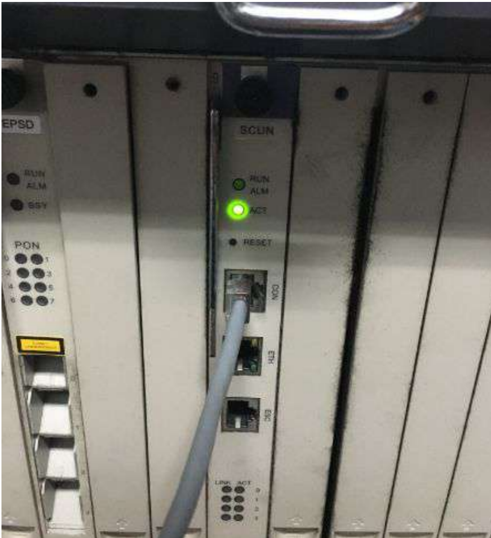
Picture 1.1 COM Port and ETH Port
